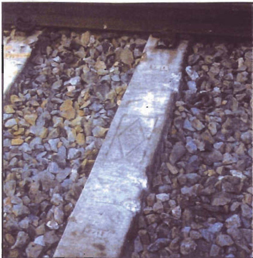
Fig.33 - Further damaged sleeper observed east of Taplow Station
